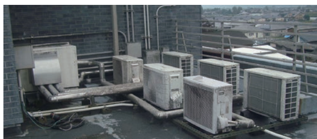
Photo 1: Volcanic ash covers the outdoor cooling units in the eruption at Mt. Aso in October 2016.
